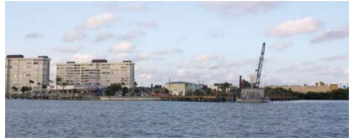
New marina being built near McDonalds at Madeira Beach
